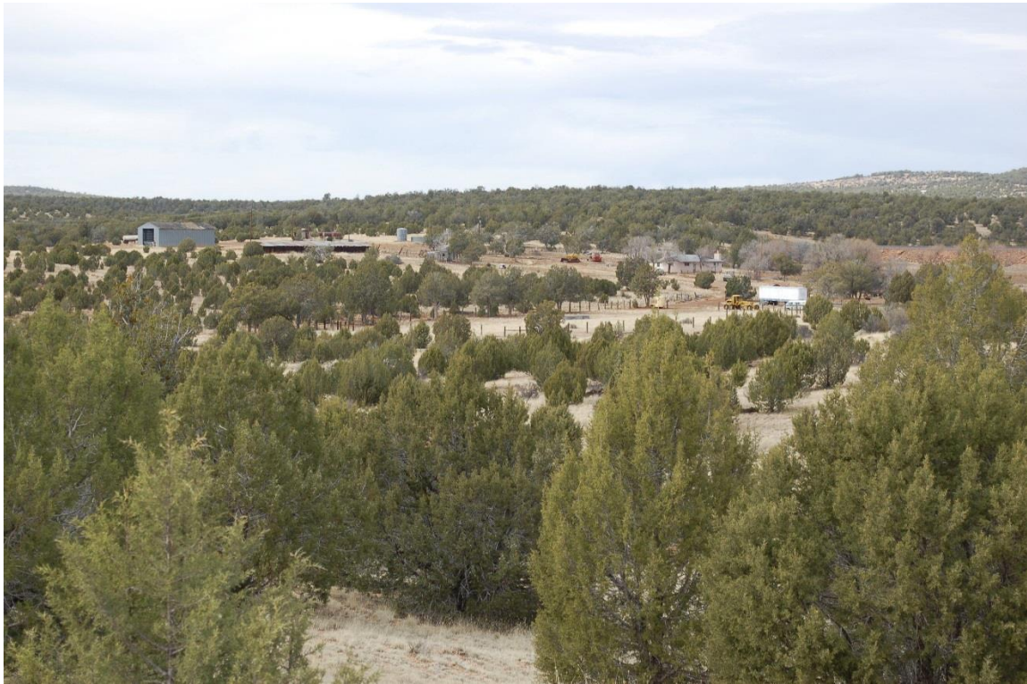
Overview of the headquarters
